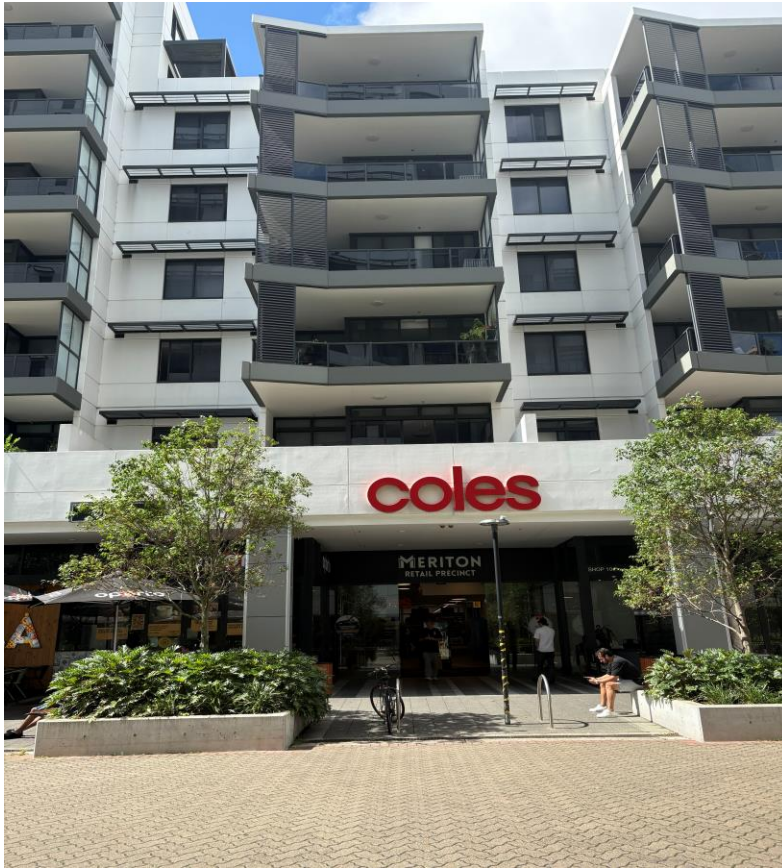
Figure 1: 782 Bourke Street, Waterloo viewed from the west
