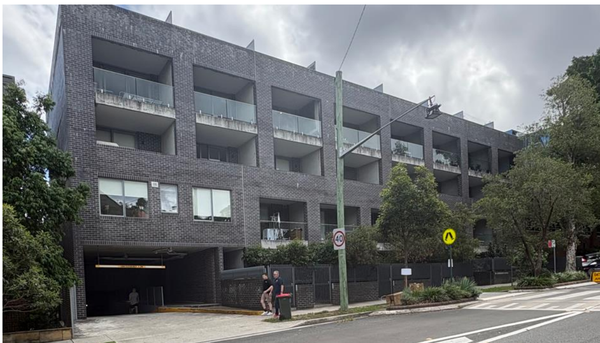
Figure 1: 12 Primrose Avenue, Rosebery, viewed from the south-east.
